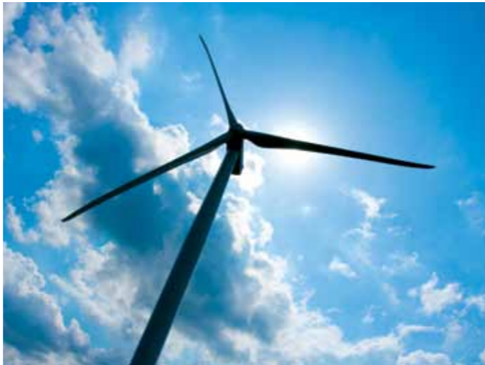
Wind electric power generators
